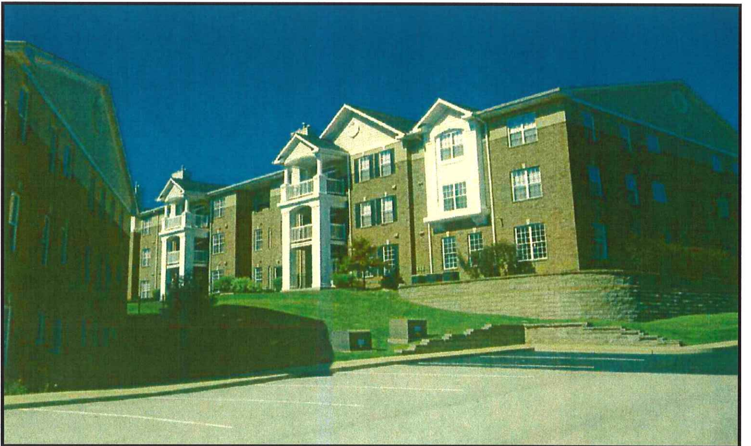
Rear view of 1175 Mill Crossing Drive (Building B) looking northwest.
