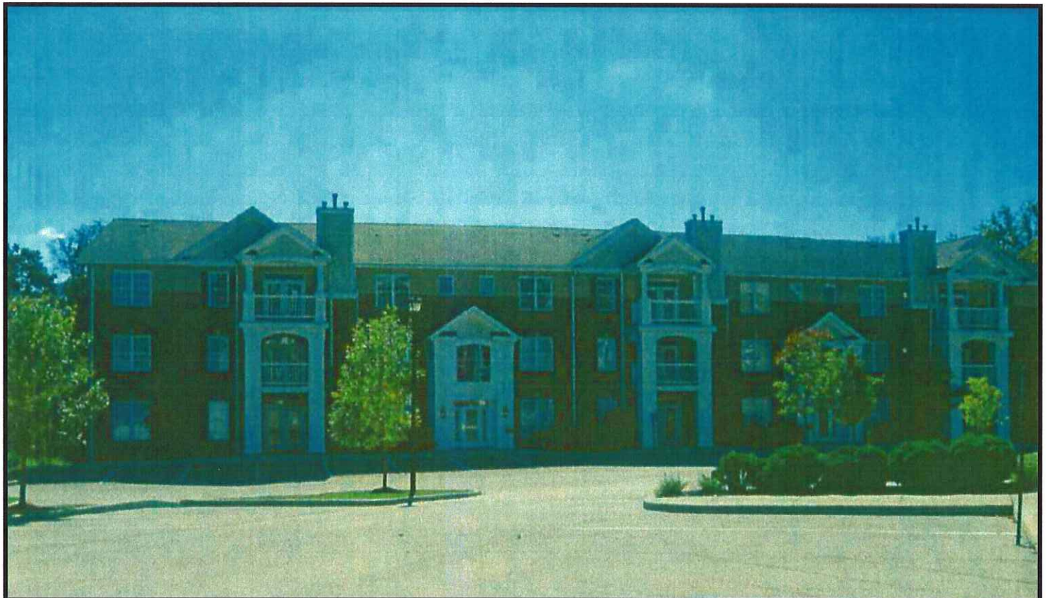
Front view of 1151 Mill Crossing Drive (Building D) looking south.
