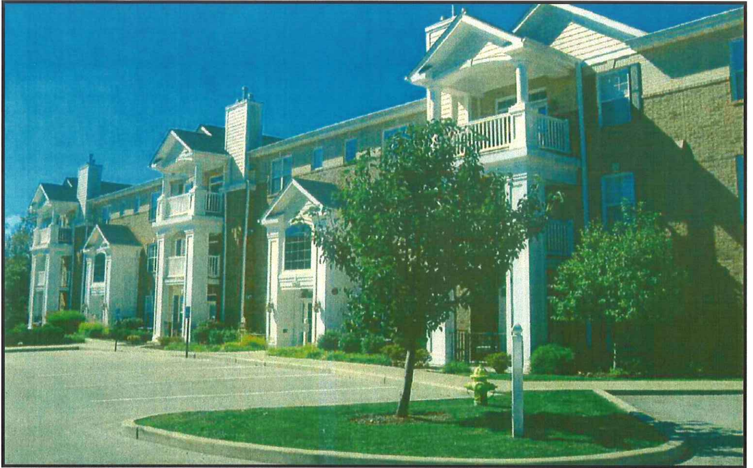
Front view of 1163 Mill Crossing Drive (Building C) looking west.
