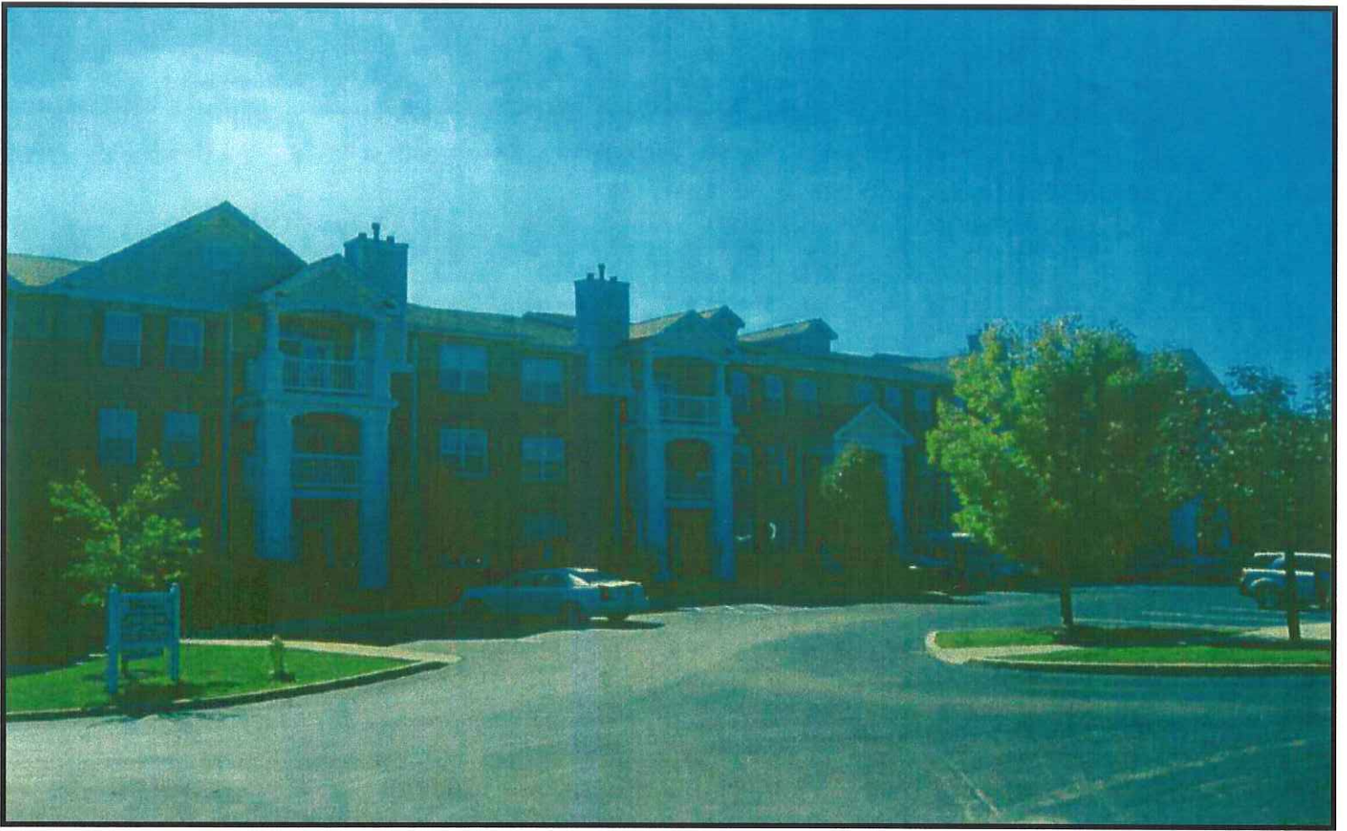
Front view of 1175 Mill Crossing Drive (Building B) looking southwest.
